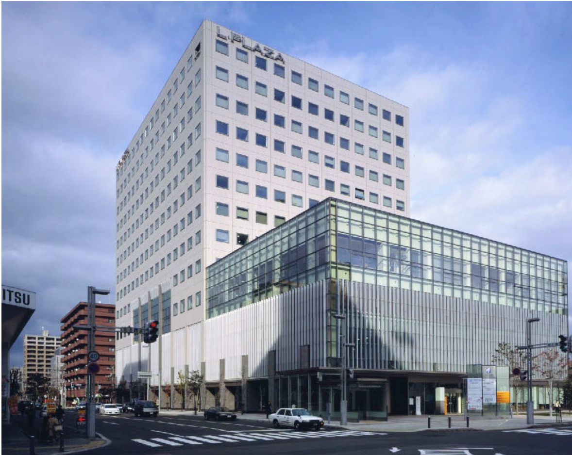
Reference Material 2 Photo of the Exterior of the Property
