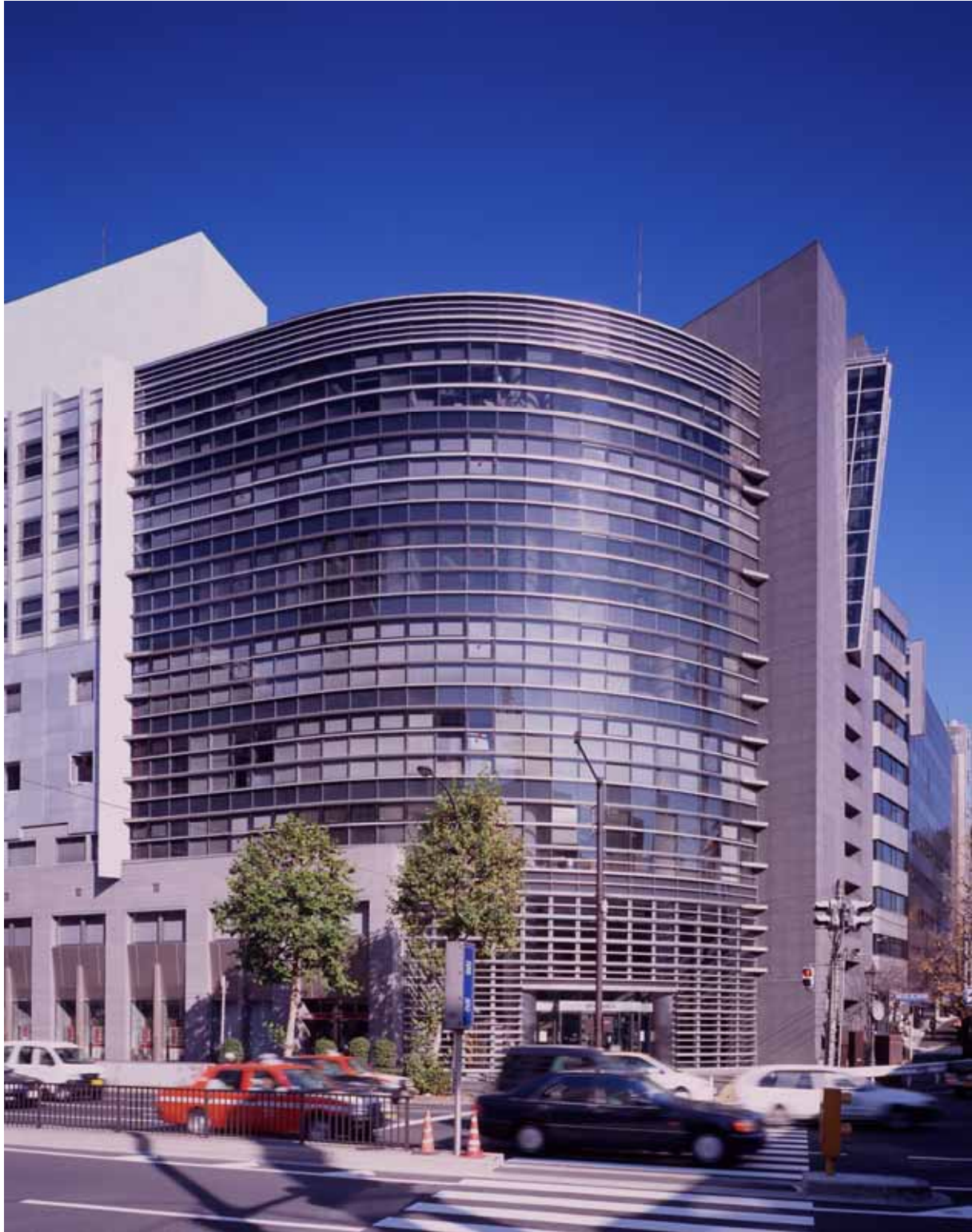
Reference Material 2 Photo of the Exterior of the Property
