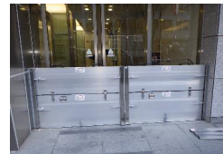
Installation of flood barriers (NBF Higashi-Ginza Square)
