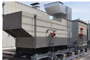
Installation of an additional emergency power generator (NBF Shibuya Garden Front)
