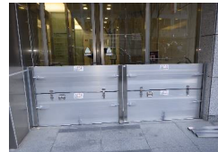
Installation of flood barriers (NBF Higashi-Ginza Square)
