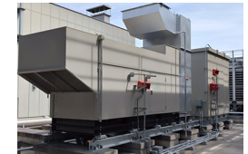
Installation of an additional emergency power generator (NBF Shibuya Garden Front)
