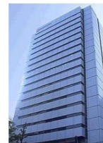
GSK Bldg. (Disposed 2017)
