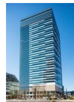
Toyosu Bayside Cross Tower (Acquired 2022-23-24)
