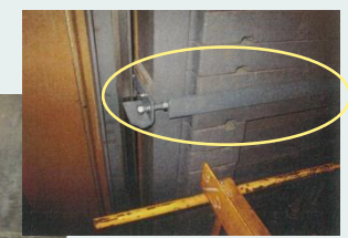
Counterweight frame reinforcement
