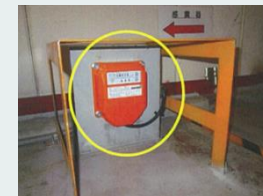
Rope misalignment stop
