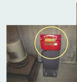
Additional earthquake sensors
