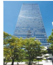
Shinjuku Mitsui Bldg. (Shinjuku-ku, Tokyo)
