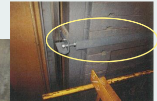
Counterweight frame reinforcement
