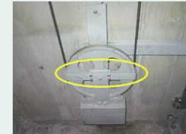
Rope misalignment stop
