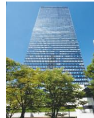
Shinjuku Mitsui Bldg. (Shinjuku-ku, Tokyo)
