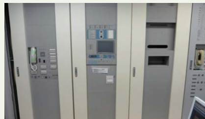
Renewal of automatic fire alarm system (Tsukuba Mitsui Bldg.)
